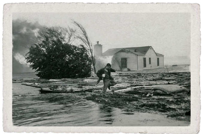
Hurricane Hazel damage, Carolina Beach, N.C., 1954. Courtesy of N.C. State Archives.
