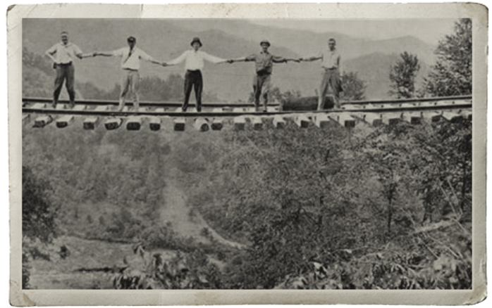
Washed-out railroad trestle over the Catawba River. Photo from "The Floods of July 1916: How the Southern Railway Organization Met an Emergency," D.H. Ramsey Library, Special Collections, University of North Carolina at Asheville.
