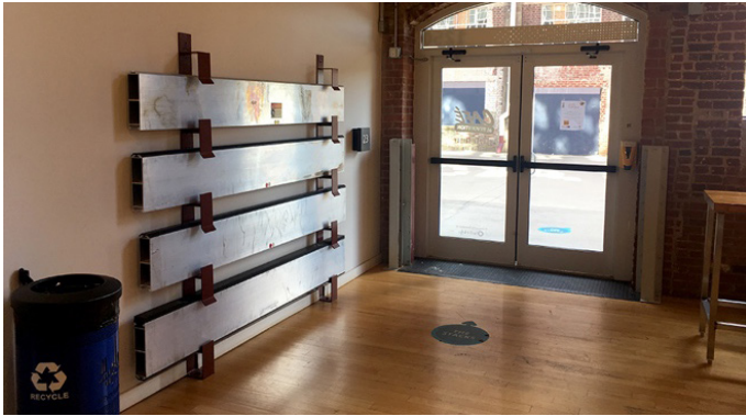
Flood logs at Revolution Mill in Greensboro, N.C., were deployed during Hurricane Florence. They held up to the rising water, which rose to 3 ft. on one side of the building. Once the danger passed, Revolution Mill stored the flood logs on custom racks, ready for quick deployment in the next storm. Courtesy of Eddie Belk, Belk Architecture.
