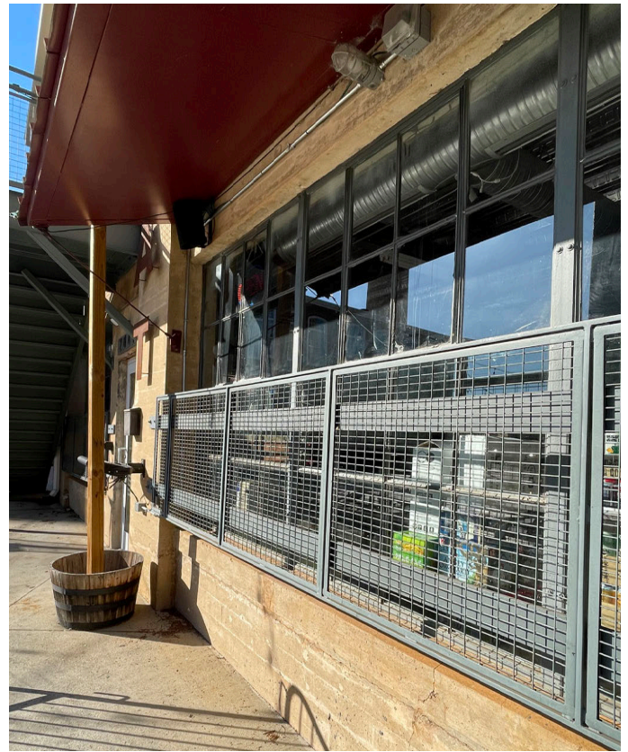
Above, grates were installed at Revolution Mill in Greensboro, N.C., to prevent flood debris from breaking windows during a flood event. Courtesy of Ramsay Leimenstoll, Architect.
