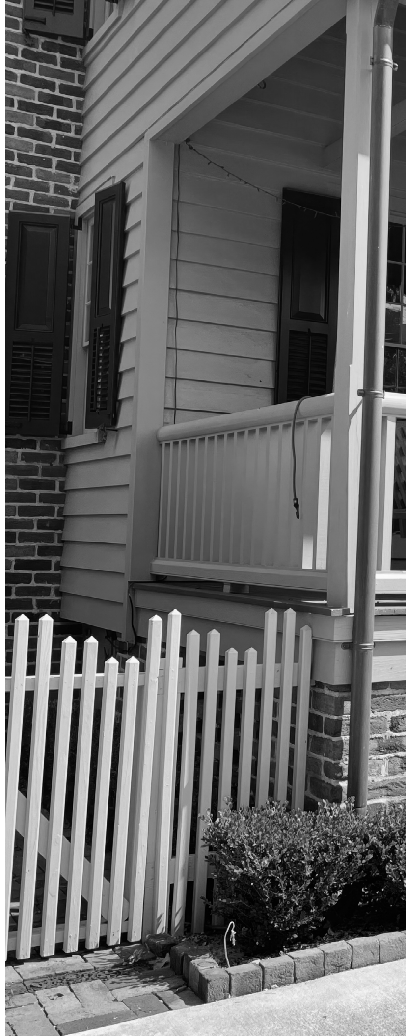
A residence in the Beaufort Historic District. Courtesy of Ramsay Leimenstoll, Architect.
