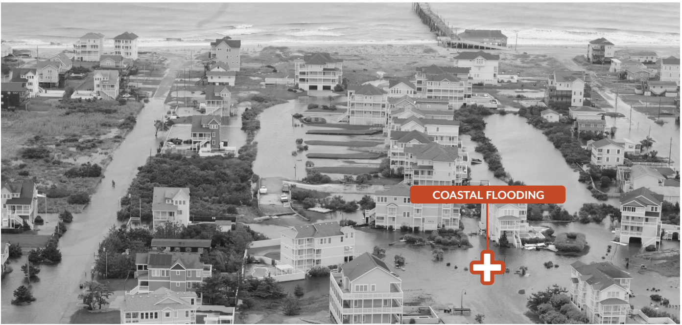
Flooding caused by Hurricane Arthur on the Outer Banks of North Carolina, July 4, 2014, photographed from a Coast Guard MH-60 Jayhawk helicopter from Air Station Elizabeth City. Courtesy of U.S. Coast Guard, Petty Officer 3rd Class David Weydert.
