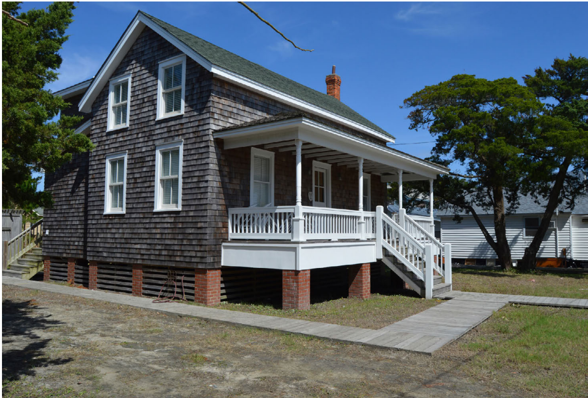
After Hurricane Matthew, this Ocracoke cottage was elevated by an additional 3'9" on new brick piers. A wide skirtboard on the porch helps minimize the perceived increase in height. Courtesy of the State Historic Preservation Office, North Carolina Department of Natural and Cultural Resources.
