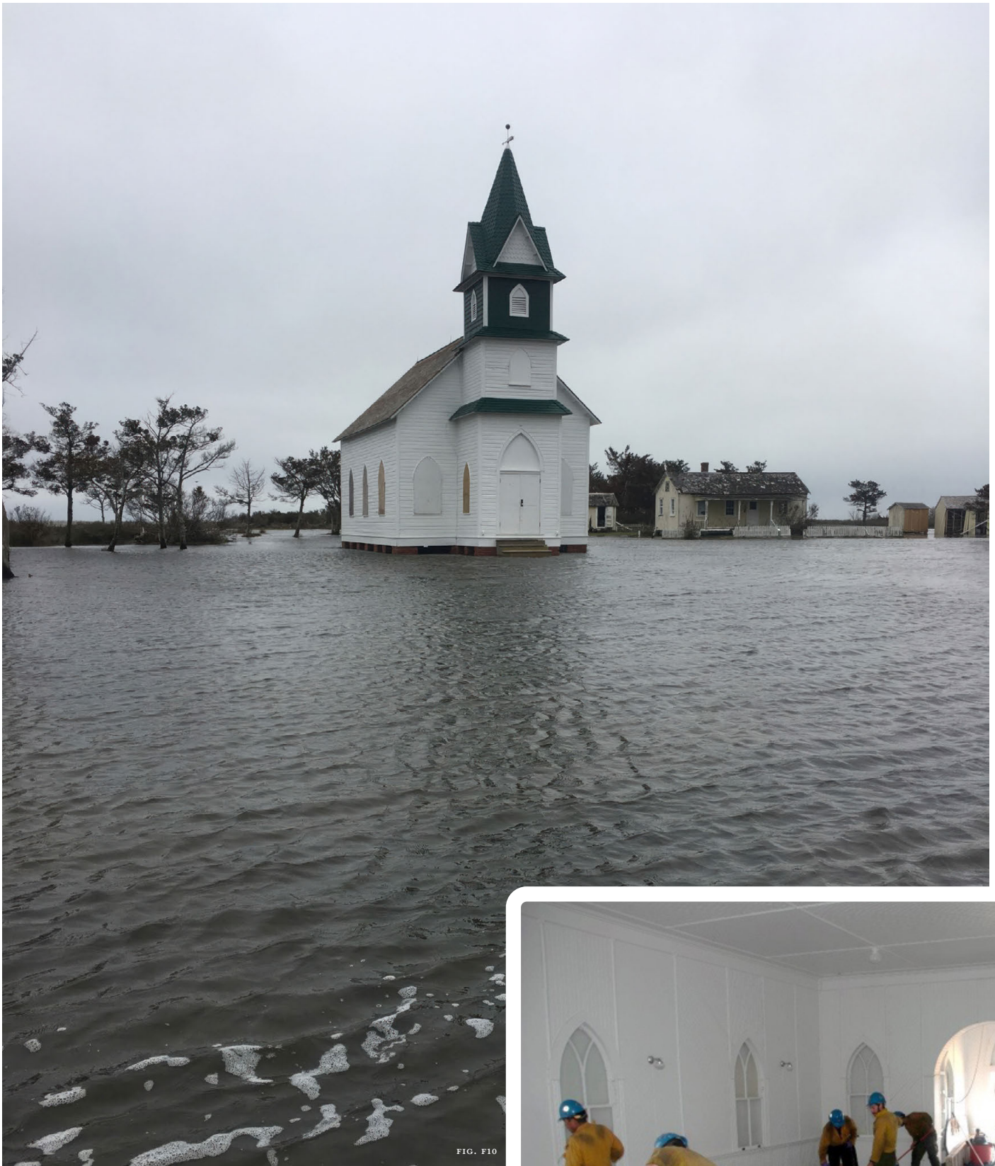
Figures F10 and F11: As flood waters receded post—Hurricane Dorian, pressure from the flood water trapped inside the Methodist Church on Portsmouth Island buckled sections of the flooring as the water sought to escape. After the interior was cleaned and dried out, the floors were repaired and trap doors were installed in the floor to provide a path for future flood waters to drain out.
