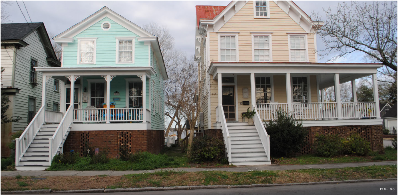
Clockwise from top left— Figure G4 : Following hurricane floods in 2004, the Biltmore Market Gardener’s Cottage in Asheville was elevated approximately 2 feet. Substantial plantings in the front yard visually screen the increased height of the foundation. Figure G5 : This Biltmore Village infill project reflects the district’s architectural character and addresses wet floodproofing principles by elevating the first floor above the established flood risk level. A raised sidewalk above the vented foundation wall helps visually minimize the increased height. Figure G6 : Although elevated approximately 5 feet above grade, the consistency of the raised foundation height and setback of these adjacent New Bern houses still maintain the character of the historic district streetscape.
