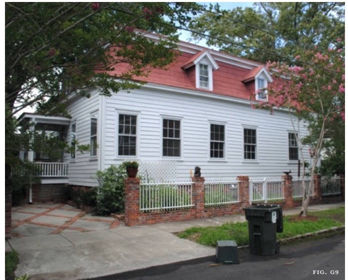
Figure G7: The foundation of this 2018 infill house in the Beaufort historic district elevates the first floor above the established flood risk level. Plantings visually screen the foundation height. Figure G8: The landscaping in front of this elevated Biltmore Village shop visually screens the raised foundation. Figure G9: When this New Bern house was moved, it was elevated above the established flood risk level. A low retaining wall with fencing set between brick piers minimizes the perceived height of the foundation along the side yard.
