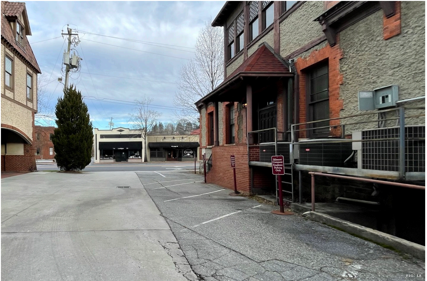
Clockwise from top left— Figure L4: HVAC units and solar panels installed far above established flood risk level on the roof of the Main Mill House are only minimally visible from distant elevated points of the Revolution Mill campus in Greensboro. Figure L5: A bank of electrical meters and panels screened from public view off the rear elevation of a property in the Beaufort Historic District were installed above the established flood risk level but are still accessible for servicing. Figure L6: New HVAC units for this elevated Ocracoke cottage were discreetly located on a raised platform aligning with the finished floor level on the side rear corner of the house. Figure L7: At St. Thomas Episcopal Church in Windsor, the mechanical unit was elevated on a secondary elevation and visually screened from view by lattice fencing. Figure L8: HVAC units and the electrical system are elevated above the established flood risk level on the side rear elevation of this commercial building in Biltmore Village.
