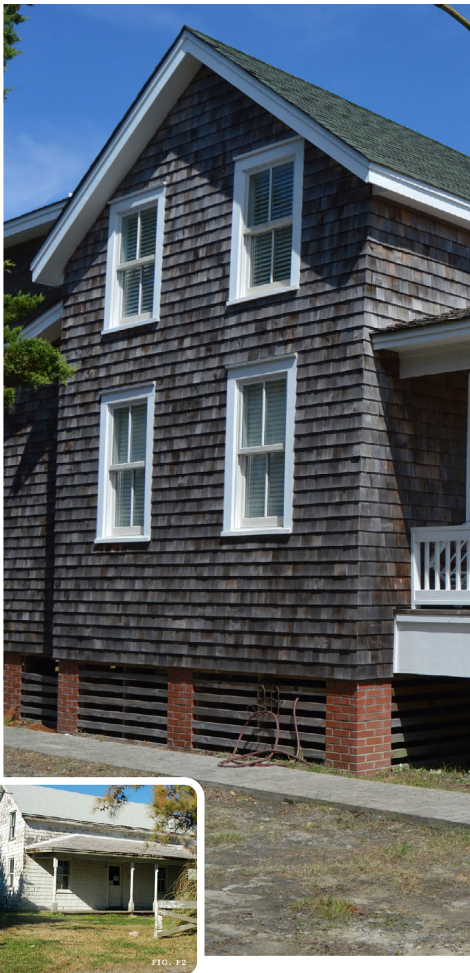
Figure F2 (inset, below left): An Ocracoke cottage before Hurricane Matthew. Figure F3 : After Hurricane Matthew, this Ocracoke cottage was elevated an additional 3’-9” on new brick piers. A wide skirtboard on the porch helps minimize the perceived increase in height. Figure F4 (inset, above right): Wooden lowered panels installed between the piers allow flood waters to flow through the cottage’s open crawl space.
