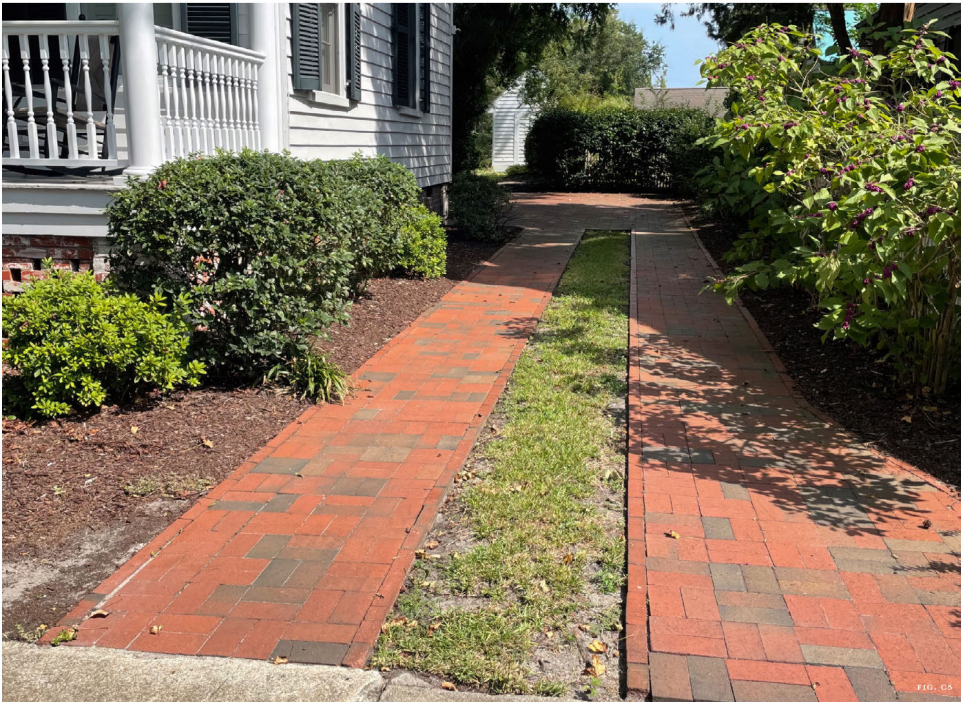
Figure C5: Two bands of brick pavers flank a planting strip to create a permeable driveway surface in Beaufort’s historic district.
