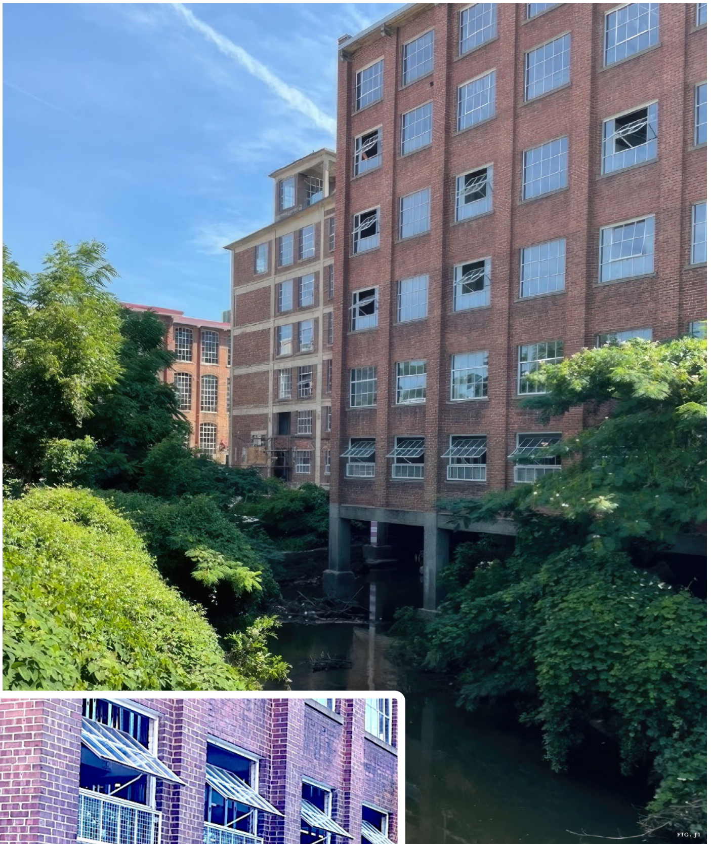
Figure J1 (above): The established flood risk level from Buffalo Creek runs 3 feet above the first floor of the Main Mill Building at Revolution Mill in Greensboro. Figure J2 (inset): To protect the building interior from floating debris during flooding, the lowest band of window lights in the original windows was replaced with laminated glass and protective metal grilles were installed in front of them.
