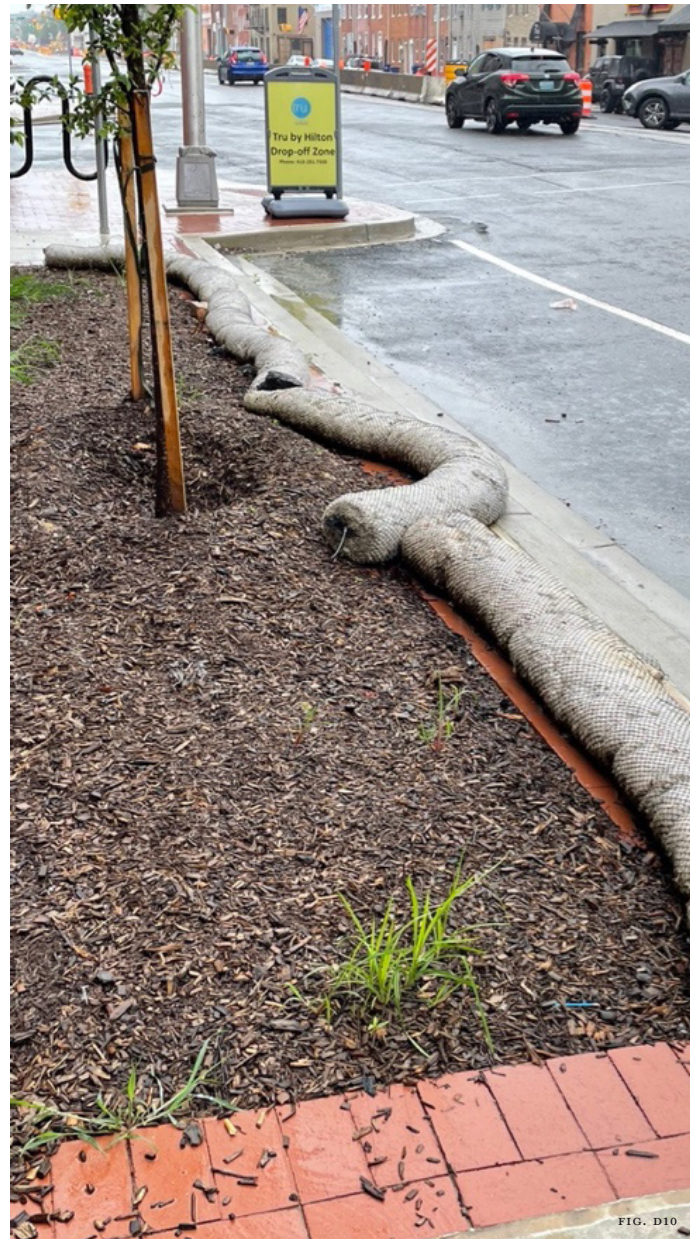
Figure D10: Sand-filled fabric tubes can help prevent loose mulch, plant matter, and debris from flowing into nearby storm sewer drains during heavy rains.
