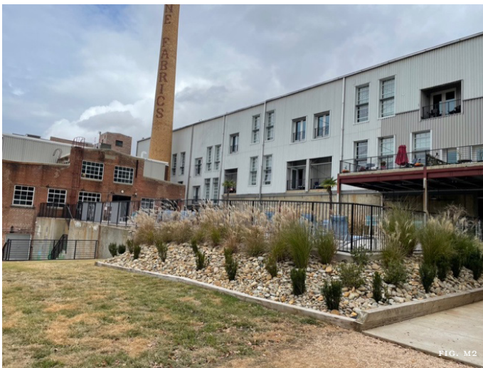
Figure M1: The massive masonry buildings at Rocky Mount Mills sited along the Falls of the Tar River were dry floodproofed when the historic complex was adapted for mixed use. Figure M2: Landscaped drainage beds buffer and separate fenced-in patio areas from the sloping Haw River site on the Granite Mill mixed-use campus.
