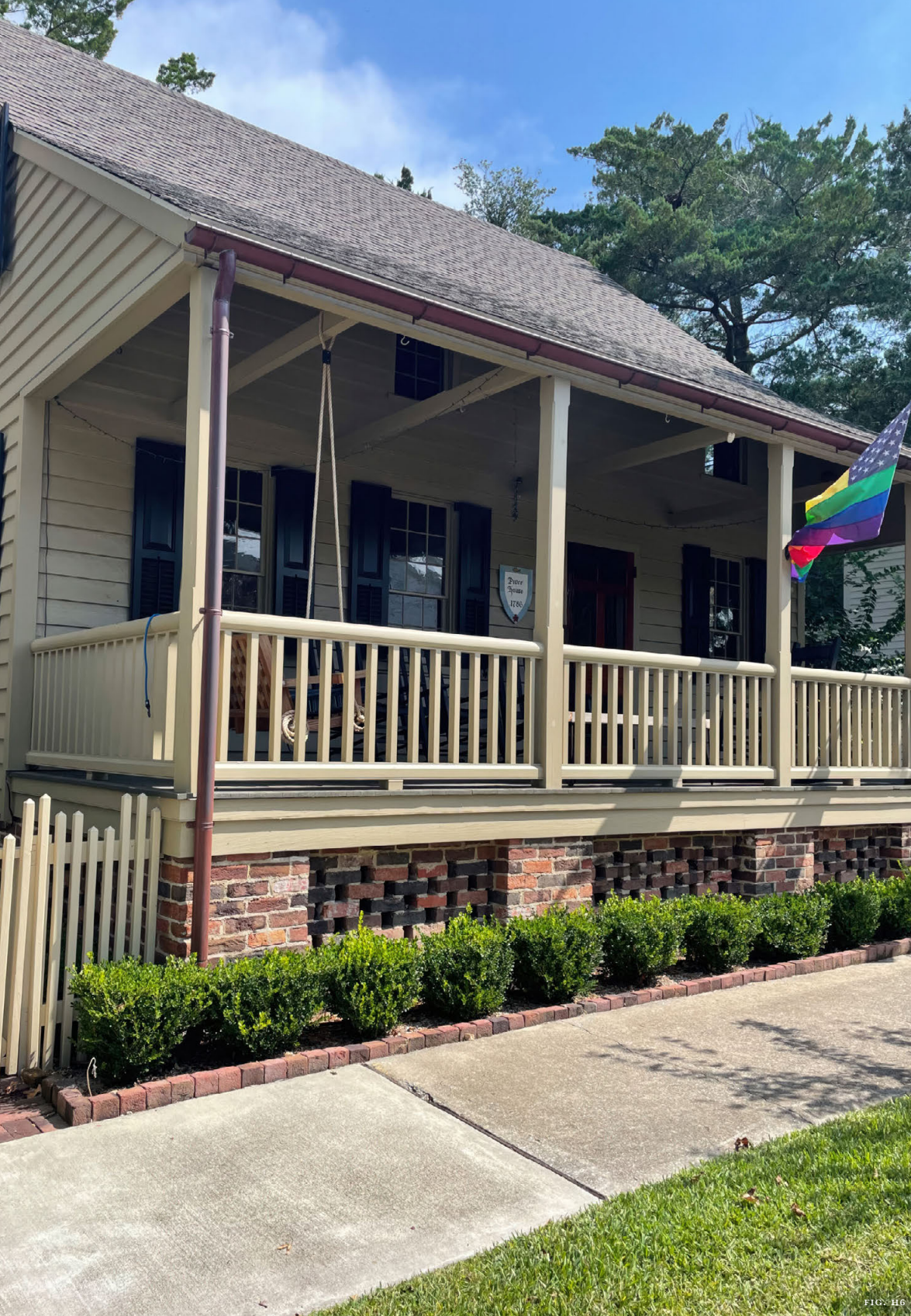
Clockwise from left— Figure H6 : A low hedge and recessed pierced brick panels minimize the visual impact of the raised brick pier foundation for this porch in the Beaufort Historic District. Figure H7 : When the Barker House in Edenton was elevated following Hurricane Isabel, flood vents were incorporated into the brick foundation. Figure H8 : New brick piers with recessed brick infill panels were used when the ca.1857 Octagon House in Hyde County was elevated approximately 2 feet to reduce water damage and improve ventilation. Figure H9 : Original, pierced brickwork vents in the foundation provide ventilation for the crawl space beneath the first floor of the Edenton Cotton Mill building. Figure H10 : When the basement of this commercial building in Biltmore Village was filled, the foundation vent opening was retained but sealed closed to prevent moisture infiltration.
