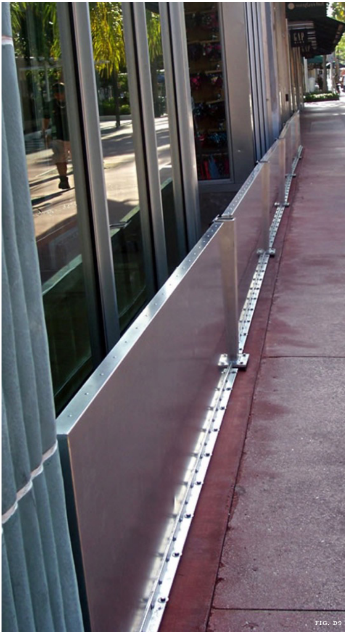
Figure D9: Temporary floodgate panels were installed to protect this commercial storefront that abuts the public right-of-way from flooding.
