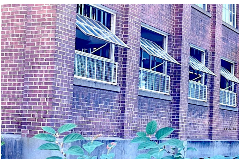
Figure J1 (above): The established flood risk level from Buffalo Creek runs 3 feet above the first floor of the Main Mill Building at Revolution Mill in Greensboro. Figure J2 (inset): To protect the building interior from floating debris during flooding, the lowest band of window lights in the original windows was replaced with laminated glass and protective metal grilles were installed in front of them.
