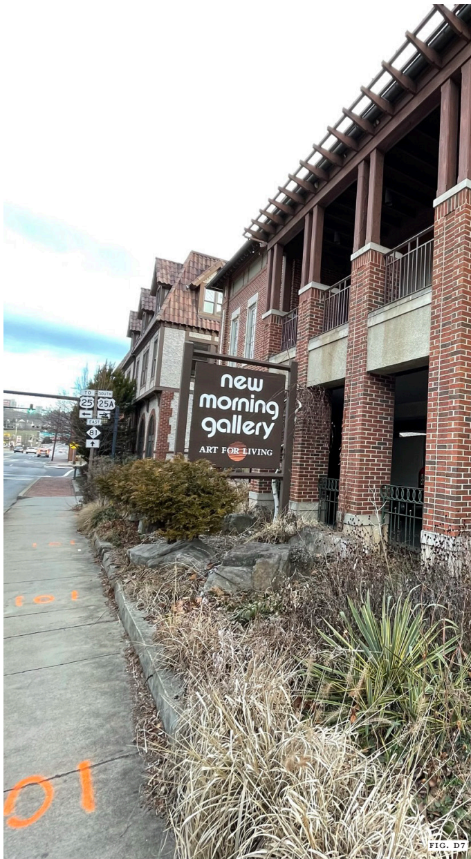
Figure D7: Raised planting beds line the public right-of-way and elevate the grade from the sidewalk to the property line of this infill building in Biltmore Village.
