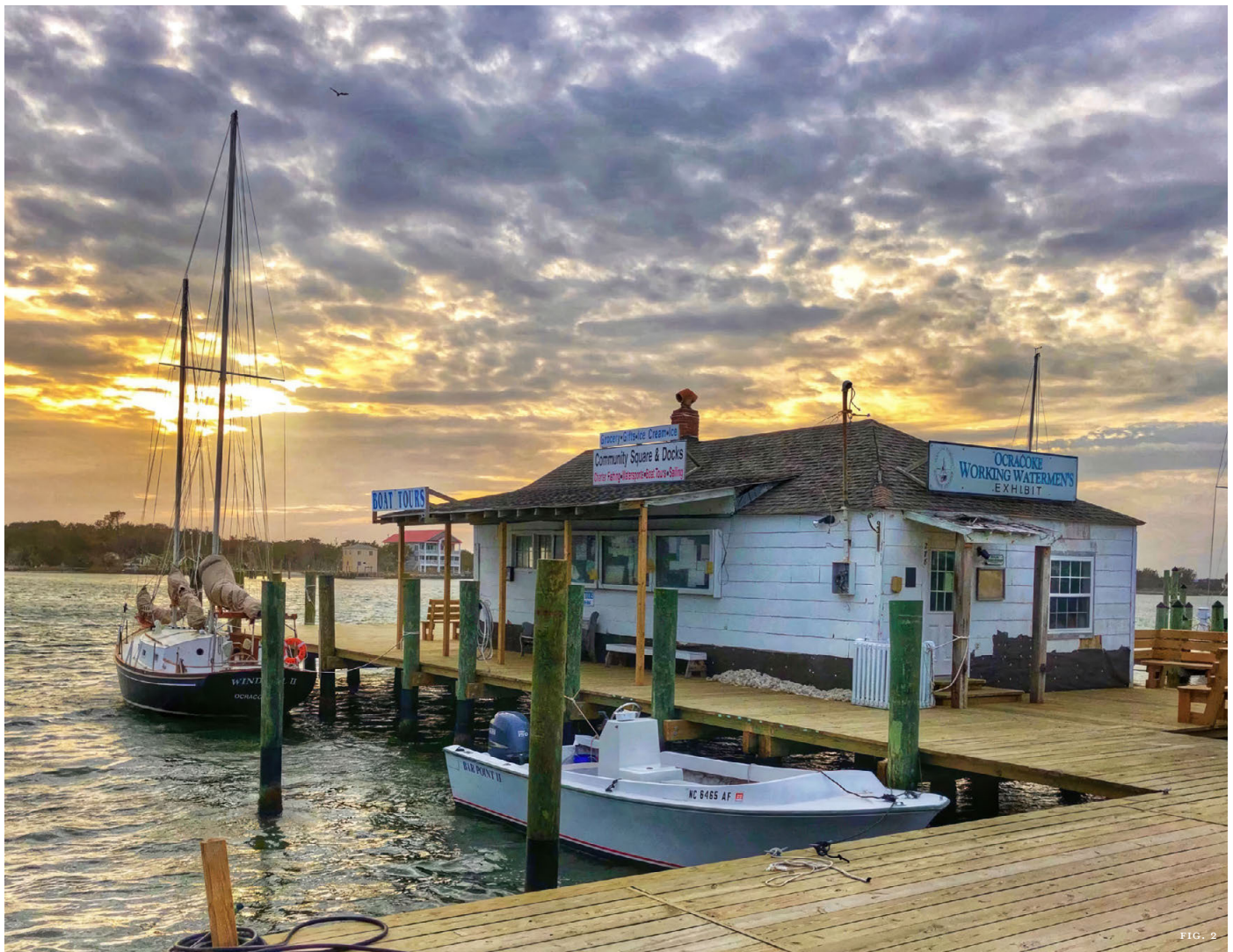
Figure 2: Damaged by high water from Hurricane Matthew, the Will Willis Fish House & Store and dock (which provides public access to the Ocracoke Harbor) were repaired and elevated 2 feet—just in time to survive Hurricane Dorian intact.
