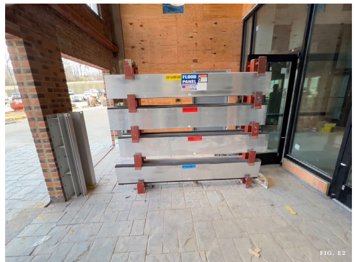
Figures E1, E2: Floodgates protect 20 doorways at Revolution Mill in Greensboro, including the entrances to the Main Mill House, where freestanding floor-mounted brackets have been installed to store the floodgate slats within the entry vestibule for easy access.
