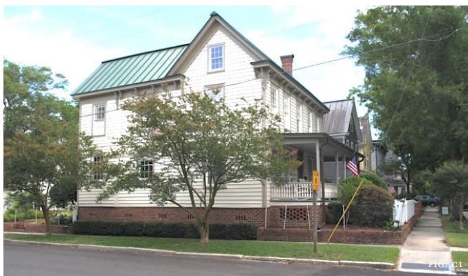
Figure C1: To minimize the visual impact when this New Bern house was elevated 5 feet above grade, fill was used to raise the front yard grade within a low retaining wall and a low hedge was added along the side elevation.
