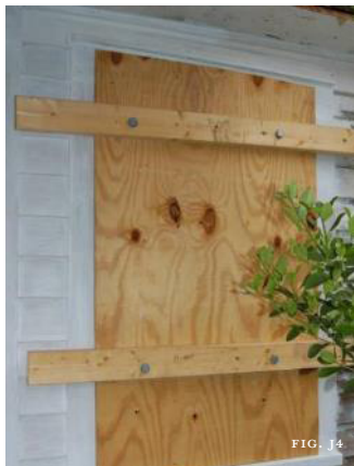
Figure J3: The operable wooden shutters on the Bellamy Mansion (foreground) and its slave quarters (background) in Wilmington are routinely closed and secured in anticipation of hurricanes to protect the windows and interior from storm damage. Figure J4: To properly secure window openings without damaging trimwork when damaged sashes are removed to make repairs, install a plywood panel over the opening and clamp 2x4s (inside and outside) with carriage bolts. Figure J5: Slide bolts at the top and bottom and a security bar across the width of the double doors in this Louisburg house reinforce them and offer extra protection of the interior during severe weather events. Figure J6: Attaching these operable shutters with longer hinges allows them to close over storm windows in this Martin County House, providing dual protection from severe weather. Figure J7: Shutters fabricated of synthetic wood with traditional details and hardware like those used on the Edmond Hoskins Store in Edenton are an appropriate resilience adaptation for historic windows in storm-prone areas.
