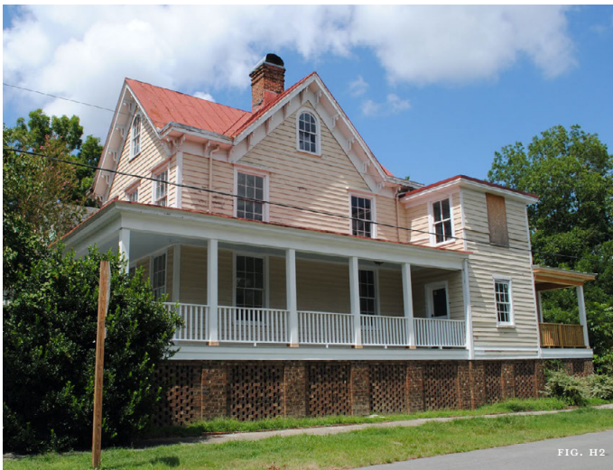
Figure H2: The new foundation of this New Bern house raises its first-floor level 5 feet above grade and approximates the configuration of its original brick piers with pierced brick infill panels that will allow future flood waters to flow through.
