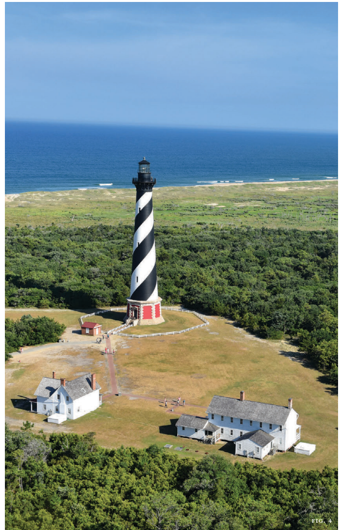
Figures 3 and 4: The Cape Hatteras Lighthouse, Principal Keeper's Quarters, and Double Keeper's Quarters were moved inland in 1999 to save them from the encroaching sea. The distance between and the orientation of the three structures are maintained at the new location to preserve the significant spatial characteristics and relationships of the historic complex.
