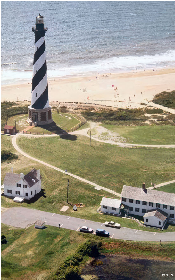
Figures 3 and 4: The Cape Hatteras Lighthouse, Principal Keeper's Quarters, and Double Keeper's Quarters were moved inland in 1999 to save them from the encroaching sea. The distance between and the orientation of the three structures are maintained at the new location to preserve the significant spatial characteristics and relationships of the historic complex.
