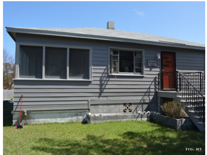
Figure H3: This mid-twentieth-century Ocracoke house was raised approximately 2 feet with fill sand, and a new concrete-block foundation with decorative block vents was constructed. A low block retaining wall defines a planting bed around the foundation and helps to minimize the change in height, as does the addition of 2 lower bands of siding that wrap the upper portion of the new foundation.
