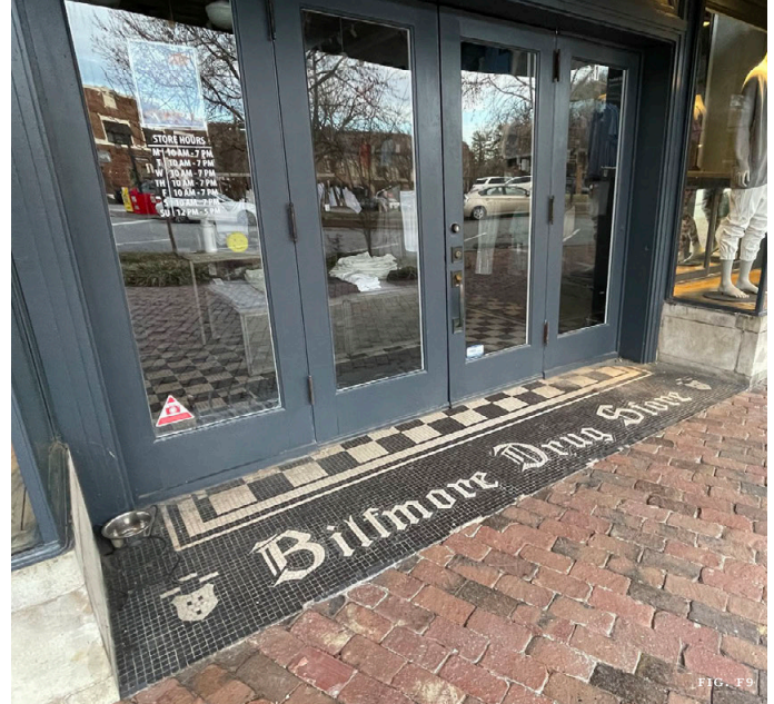
Figure F8: Some basement areas in this commercial block that abut the public right-of-way in Biltmore Village were filled in, and some wooden floors were replaced with concrete to protect them from future flood damage. Figure F9: Fortunately, the resilient ceramic tiles on this corner building have survived multiple floods intact.
