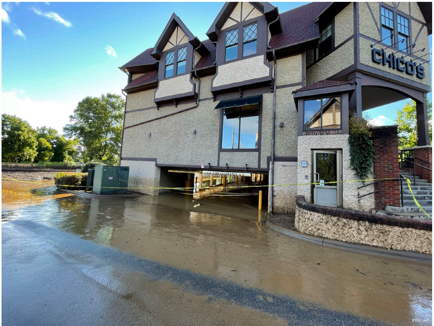
Figure A8: The lower-level parking deck of this Biltmore Village infill building also functions as a holding area for flood water.
