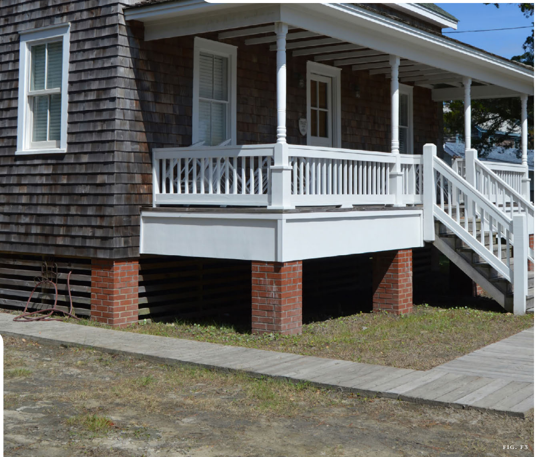
Figure F2 (inset, below left): An Ocracoke cottage before Hurricane Matthew. Figure F3 : After Hurricane Matthew, this Ocracoke cottage was elevated an additional 3’-9” on new brick piers. A wide skirtboard on the porch helps minimize the perceived increase in height. Figure F4 (inset, above right): Wooden lowered panels installed between the piers allow flood waters to flow through the cottage’s open crawl space.
