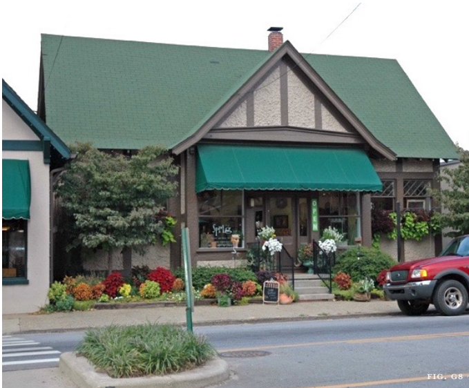
Figure G7: The foundation of this 2018 infill house in the Beaufort historic district elevates the first floor above the established flood risk level. Plantings visually screen the foundation height. Figure G8: The landscaping in front of this elevated Biltmore Village shop visually screens the raised foundation. Figure G9: When this New Bern house was moved, it was elevated above the established flood risk level. A low retaining wall with fencing set between brick piers minimizes the perceived height of the foundation along the side yard.
