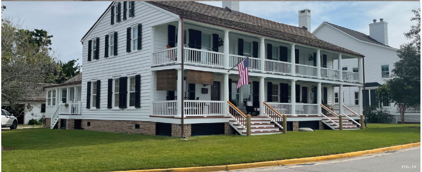
Figure 14: View of the Duncan House in Beaufort prior to being elevated. Figure 15: The Duncan House was elevated on a new brick foundation and porch piers — without significantly impacting its historic character or the character of the district streetscape. The foundation vents between the porch piers were painted a dark color to make them visually unobtrusive and the porch steps incorporate traditional cutouts in the risers, allowing water to drain off and enhancing ventilation beneath them.
