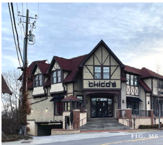
Figure M6: This Biltmore Village infill project incorporates wet floodproofing principles, with a wet basement parking area and lobby space on the lower level and retail spaces on the second floor above the established flood risk level. Figure M7: Given its proximity to the French Broad River and its relatively low site, the historic Madison County Courthouse's location in downtown Marshall is vulnerable to flash flooding. Figure M8: Metal stanchions installed to hold temporary floodgates flank this utilitarian roll-up door to a brewery's storage area on a rear elevation at Rocky Mount Mills.
