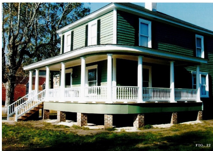
Figure 11: In Burgaw, when this house was elevated 30 inches, the wraparound porch was elevated on new brick piers. Figure 12: The original porch columns and railings were retained, and the steps were extended to accommodate the increased porch height.
