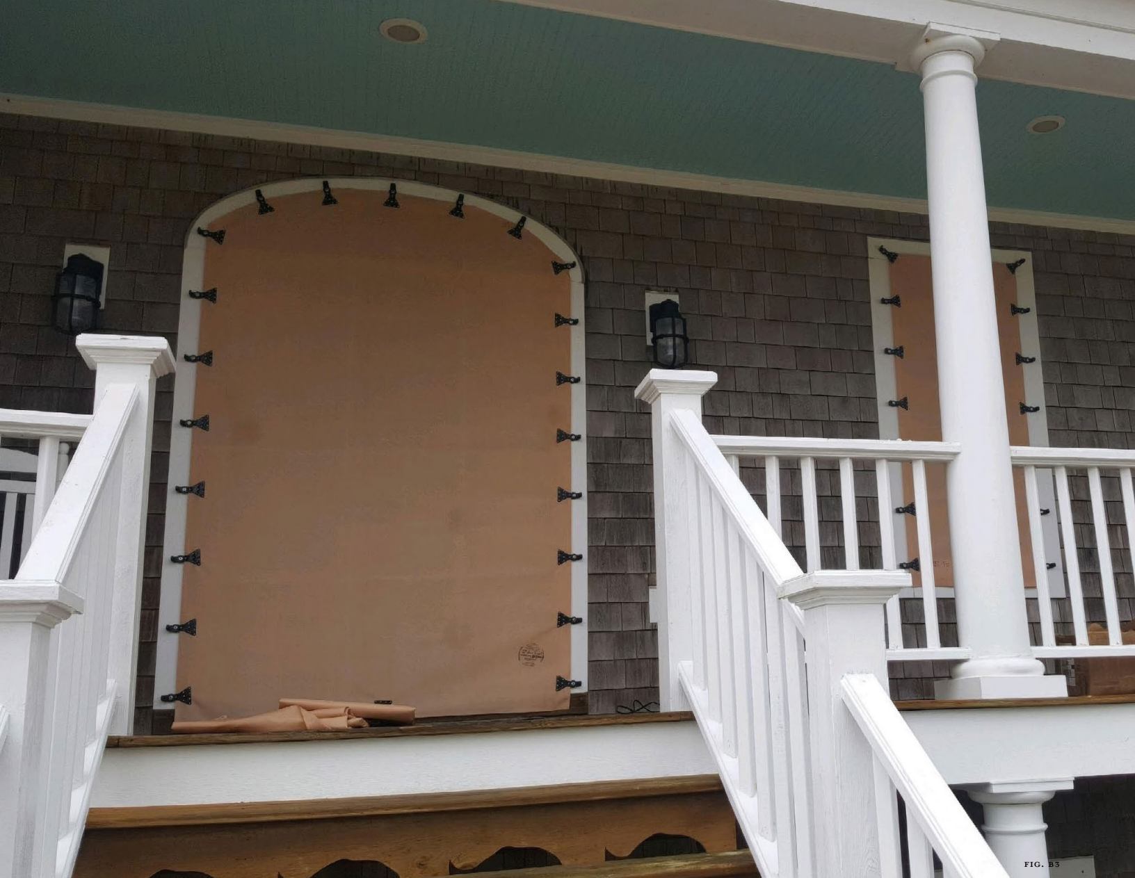
Figure B3: On this Morehead City residence, high tensile–strength hurricane fabric panels, held in place with metal clips, offer temporary protection to door and window openings from high-velocity winds and flying debris.
