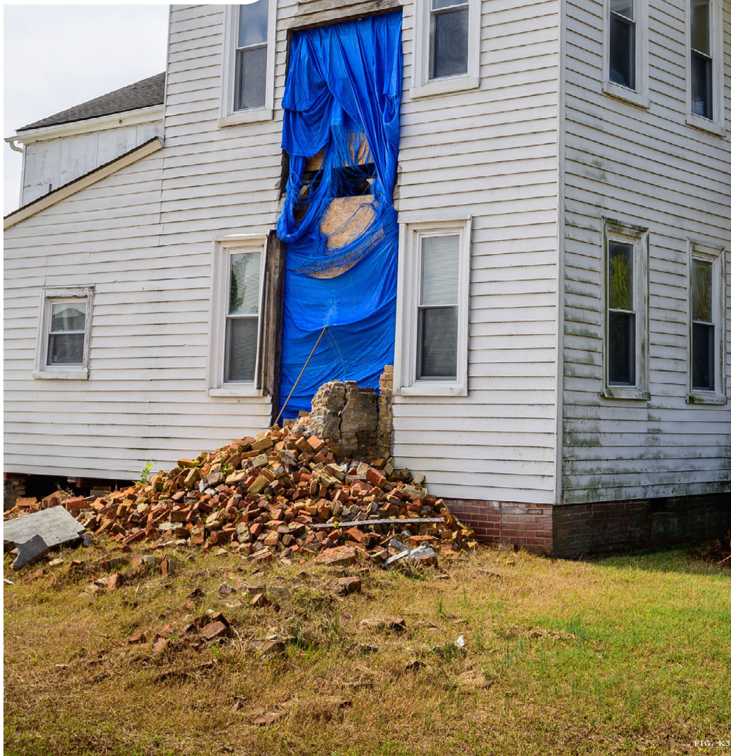
Figure K3: The east chimney of the 1835 William T. Smith House collapsed due to the impact of Hurricane Florence.
